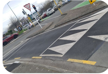
Tie ramp into channel
