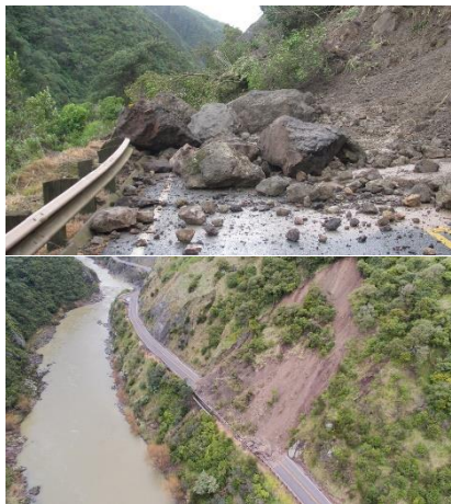
Debris from slip that occurred on 23 July 2017
