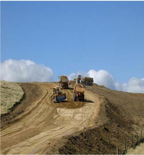
The roads were constructed to 10 meter formation widths to allow crane access and the carriage of long tower and blade units. Roads connected to the main road were sealed.
