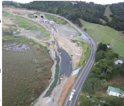
*RW02: Reinforced slope RW02 under construction in the centre of the picture*
