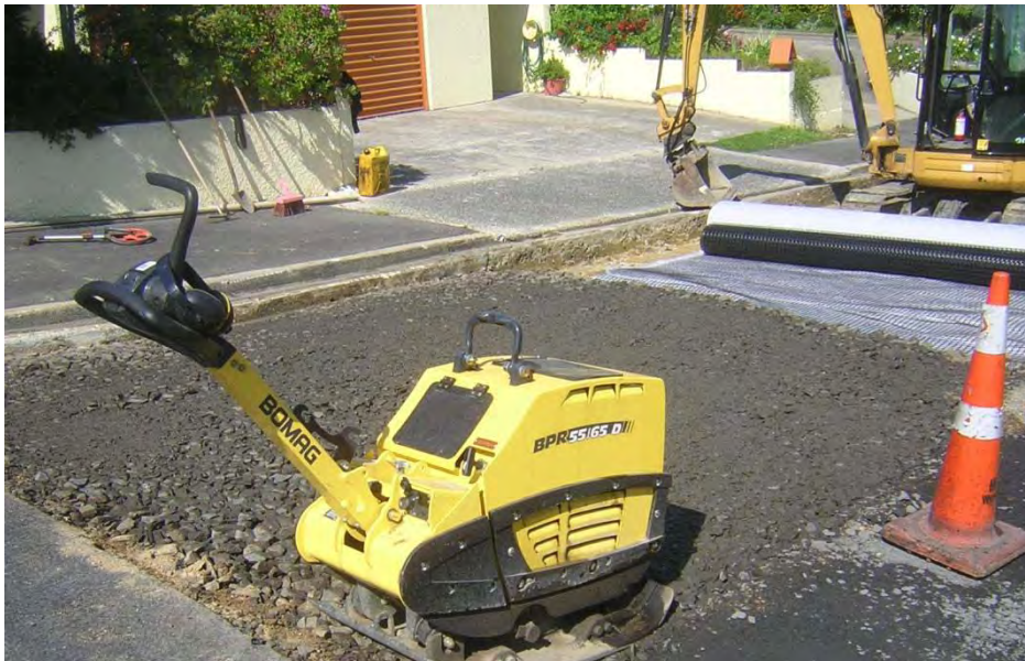
Compacted with 480kg reversible plate
