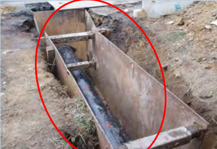
Launch pit with shoring
