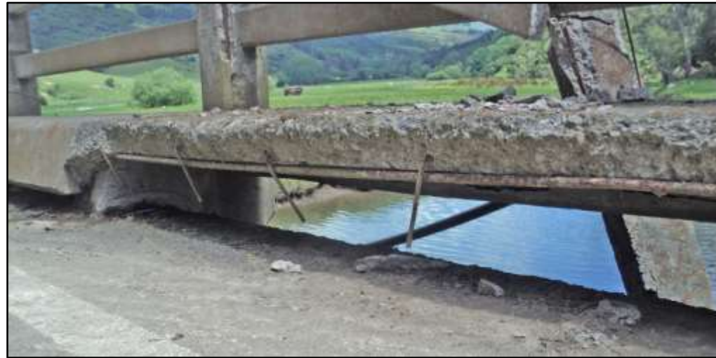
Typical damage/spalling issues
