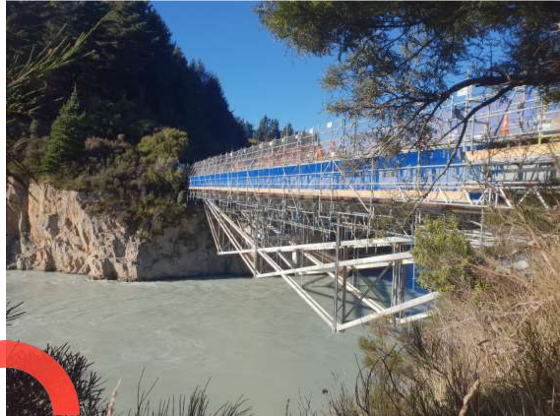
Scaffolding of Structure (Source: Downer NZ)
