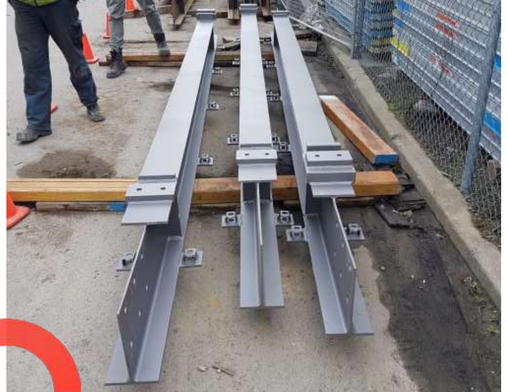
Steel UB transoms in storage yard (Source: Downer NZ)
