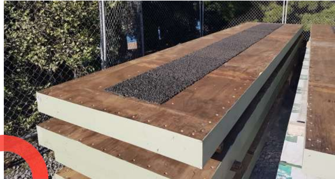
BRP road patch on Laminated Timber Panel
