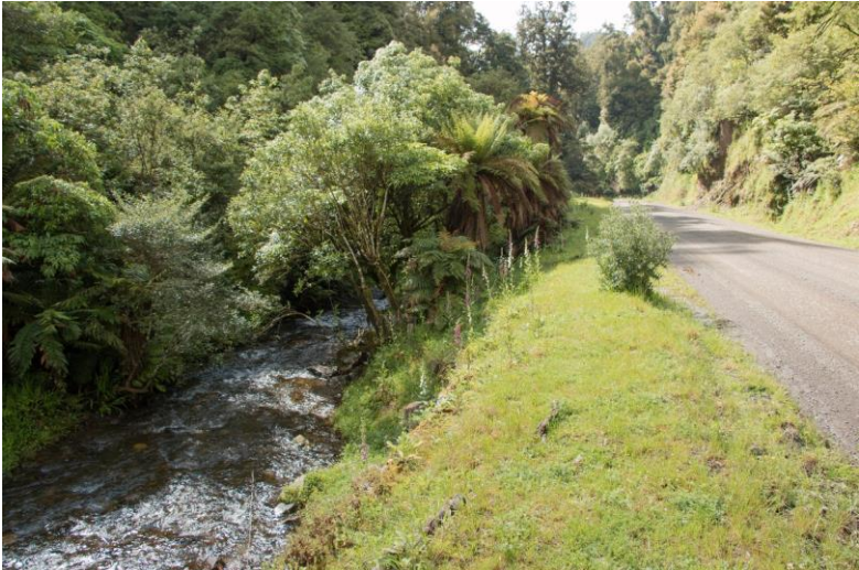
Ruatāhuna Road at Mangapae Stream
