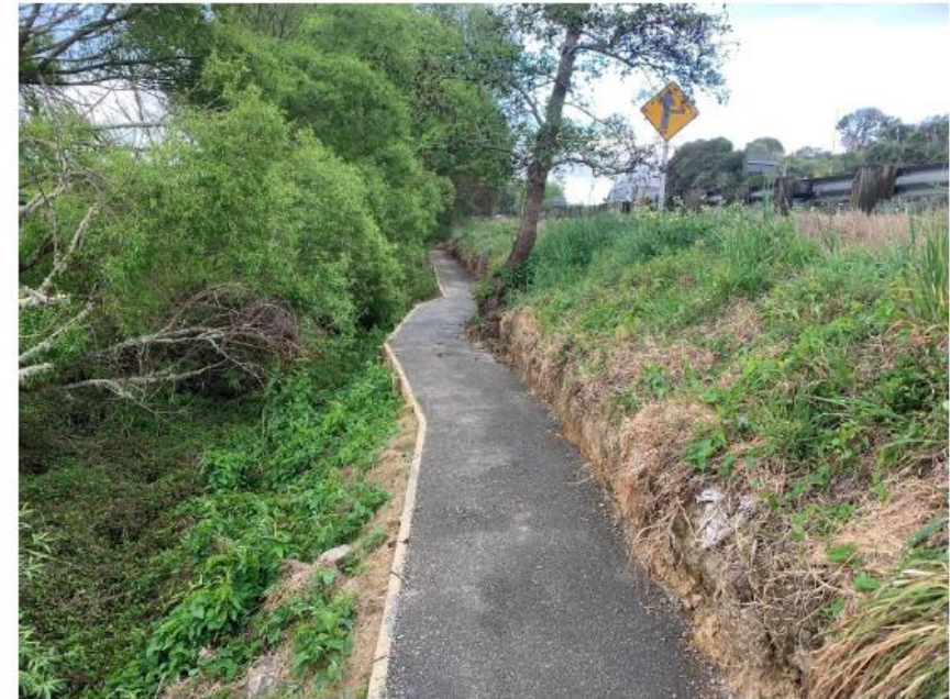
S10 surfacing. Width up to 1.4m
